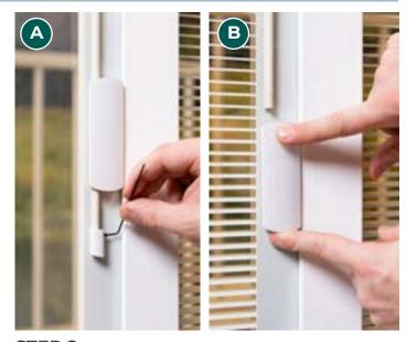
STEP 2: Remove the end cap set screw
