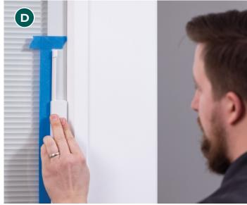
STEP 2.2: Align and Apply New Operator and Track
