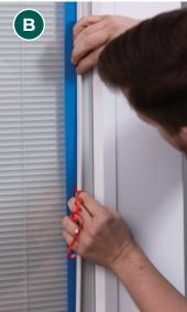
STEP 2: Align and Apply New Operator and Track
