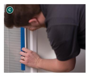
STEP 2.1: Align and Apply New Operator and Track
